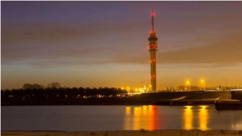
Our primary datacenter is housed in the Media tower of Cellnex in Lelystad (NL)
